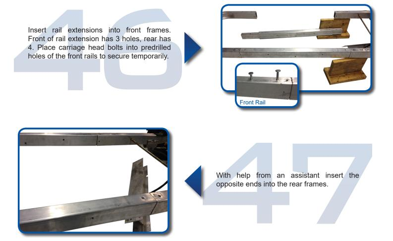
NOTE: Once rails and frames are joined, line up the 6 drilled holes from step 43 using a 21/64" bit, drill through bottom of the frame.
